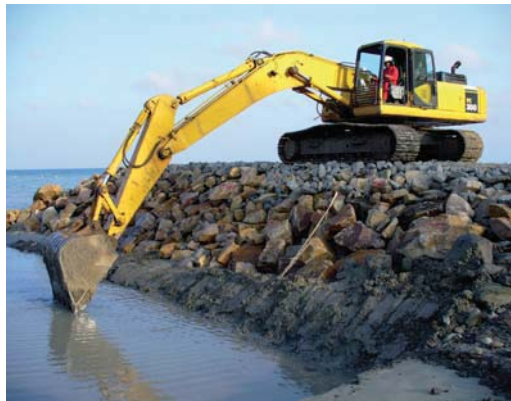
Construction embankment dam
